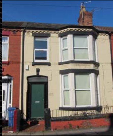
49 Portman Road L15 2HH
